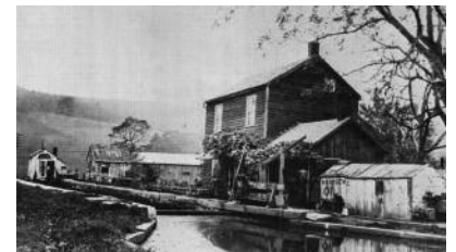
Lock 7 West near New Village. The store at the far end of the lock sold goods to boatmen including homemade pies & bread. It was known for many years as "Gardner's" Lock and also as "Fresh Bread" Lock. The sign on the store reads "Homemade Potato Bread."
